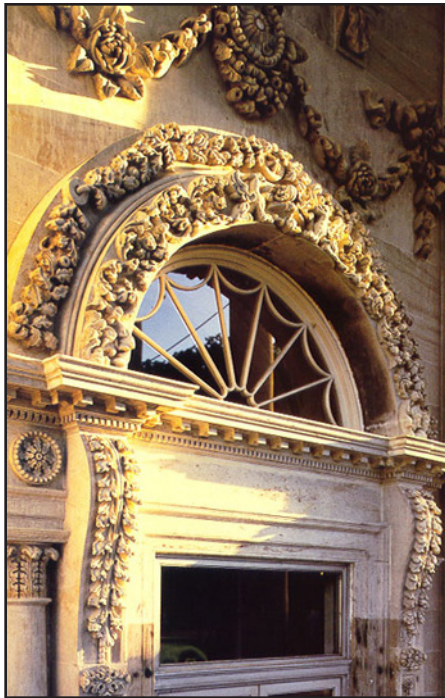
North front with 42 layers of white paint removed. Richard Cheek, The White House
