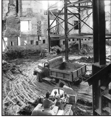
A bulldozer digs out two new basement levels for the White House in 1950. Abbie Rowe, National Park Service
